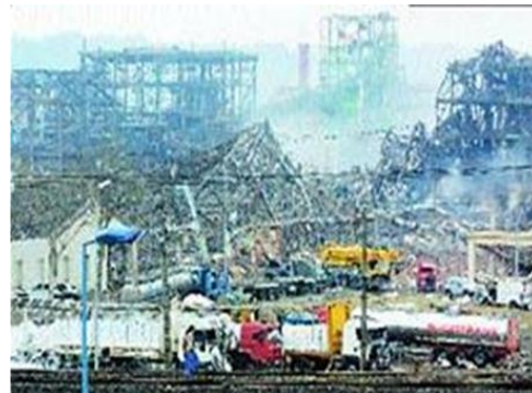
Toulouse Site Damage
